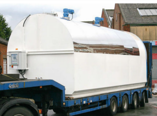
30,000 litre Bunded Tank ready for re-location.
